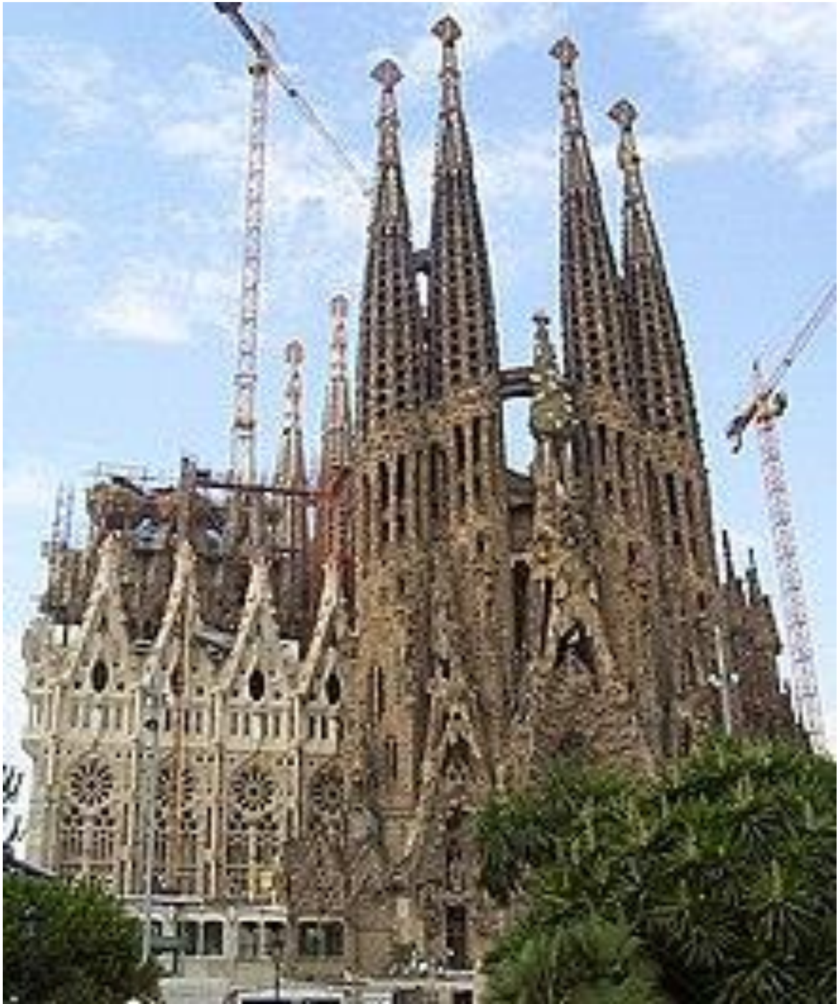
Sagrada Famiflia under construction
